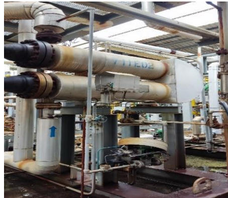
Gambar 2. Jalur H 2 Masuk Feed Natural Gas
